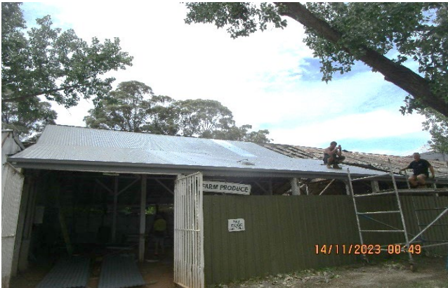
Martin, Tony and Max - Weber Constructions strip and replace iron and roof frame section at a time.
