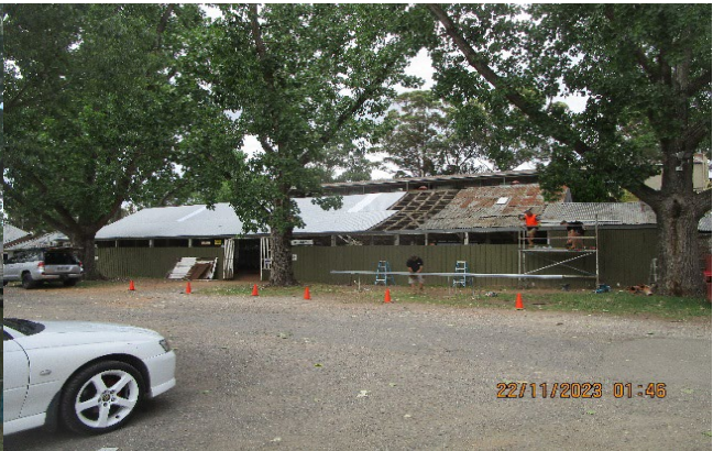
Martin, Tony and Max - Weber Constructions strip and replace iron and roof frame section at a time.
