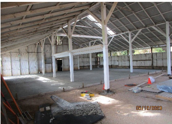
Stage 1 slab down. Slab Stage 2 site excavated, underlay down, mesh about to be fixed in place.
