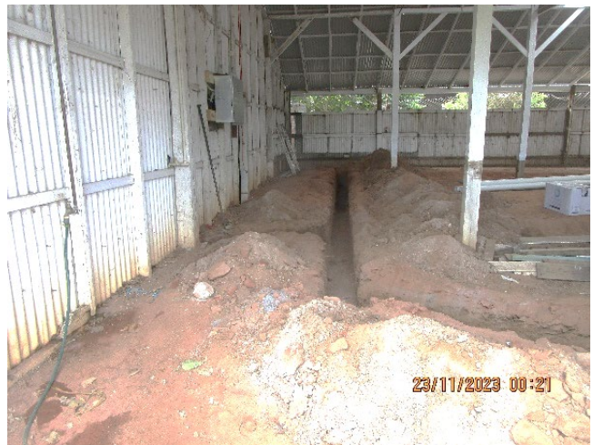
Internal drainage line runs the full length and width of the pavilion.
