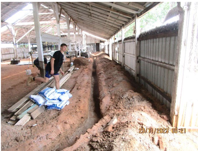
Internal drainage line runs the full length and width of the pavilion.
