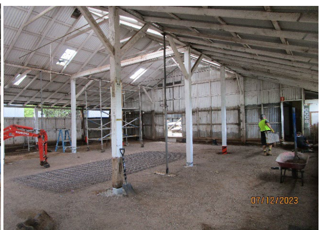
Stage 1 slab down. Slab Stage 2 site excavated, underlay down, mesh about to be fixed in place.
